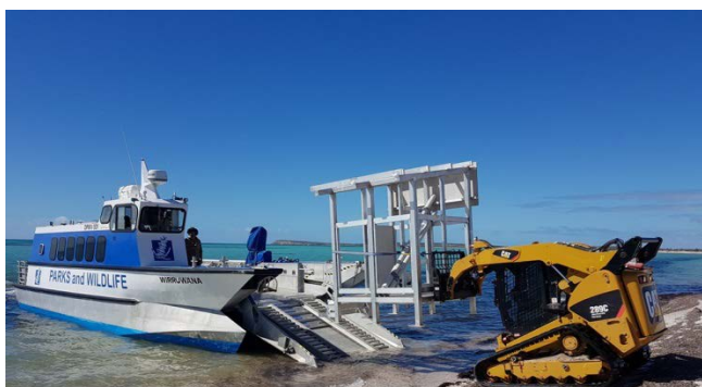
Prefabricated toilet structure being unloaded at Herald Bay.
